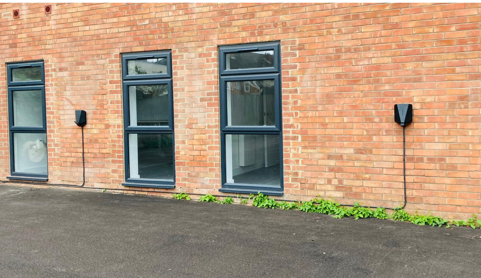
Installation of 2x Easee EV charging points 7Kw. This type of installation allows us to install additional charging points at a later stage, if needed.
