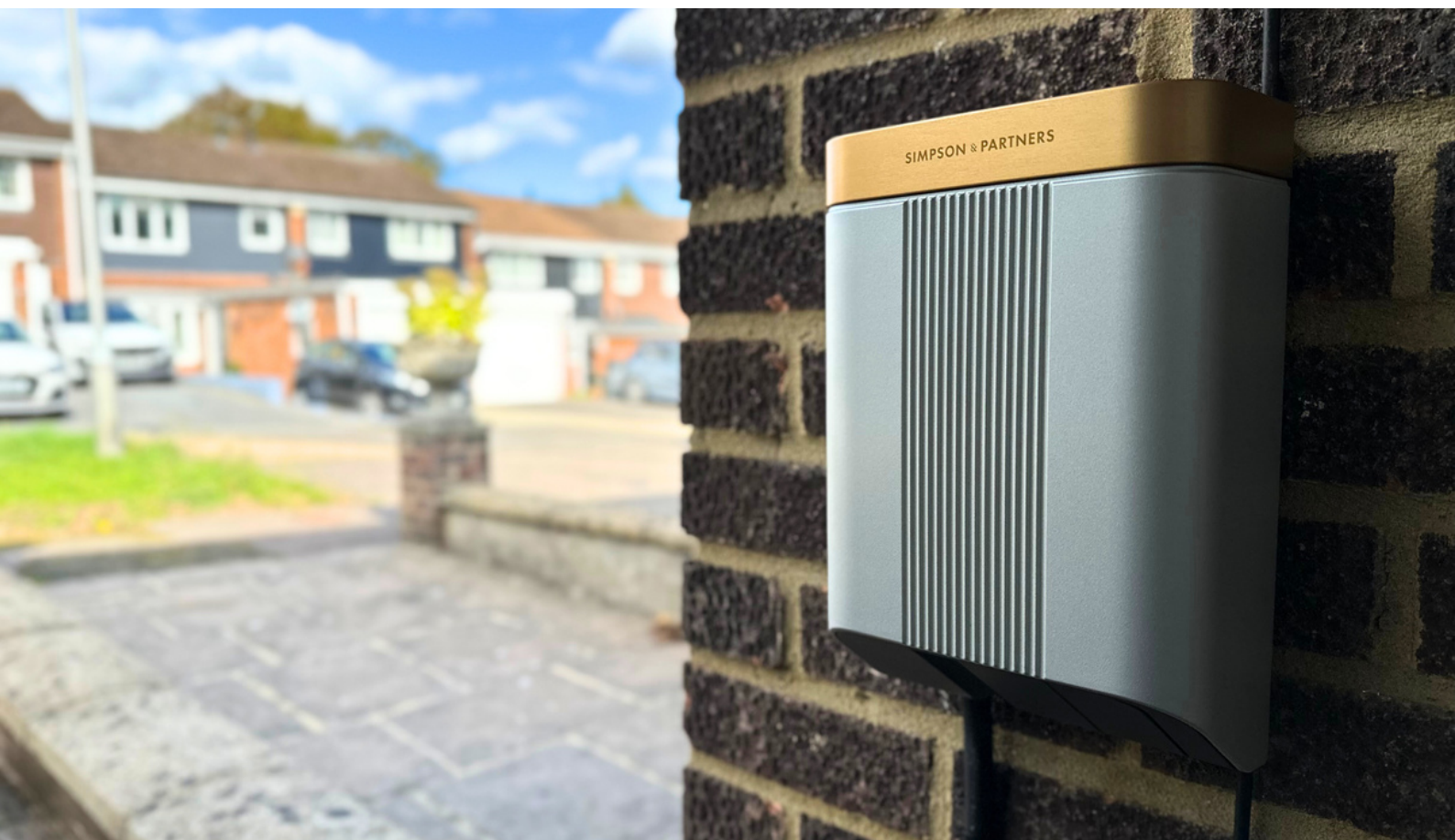
Another domestic installation of 1x EV single phase charging point. This type of installation supports PV solar panels connectivity.
