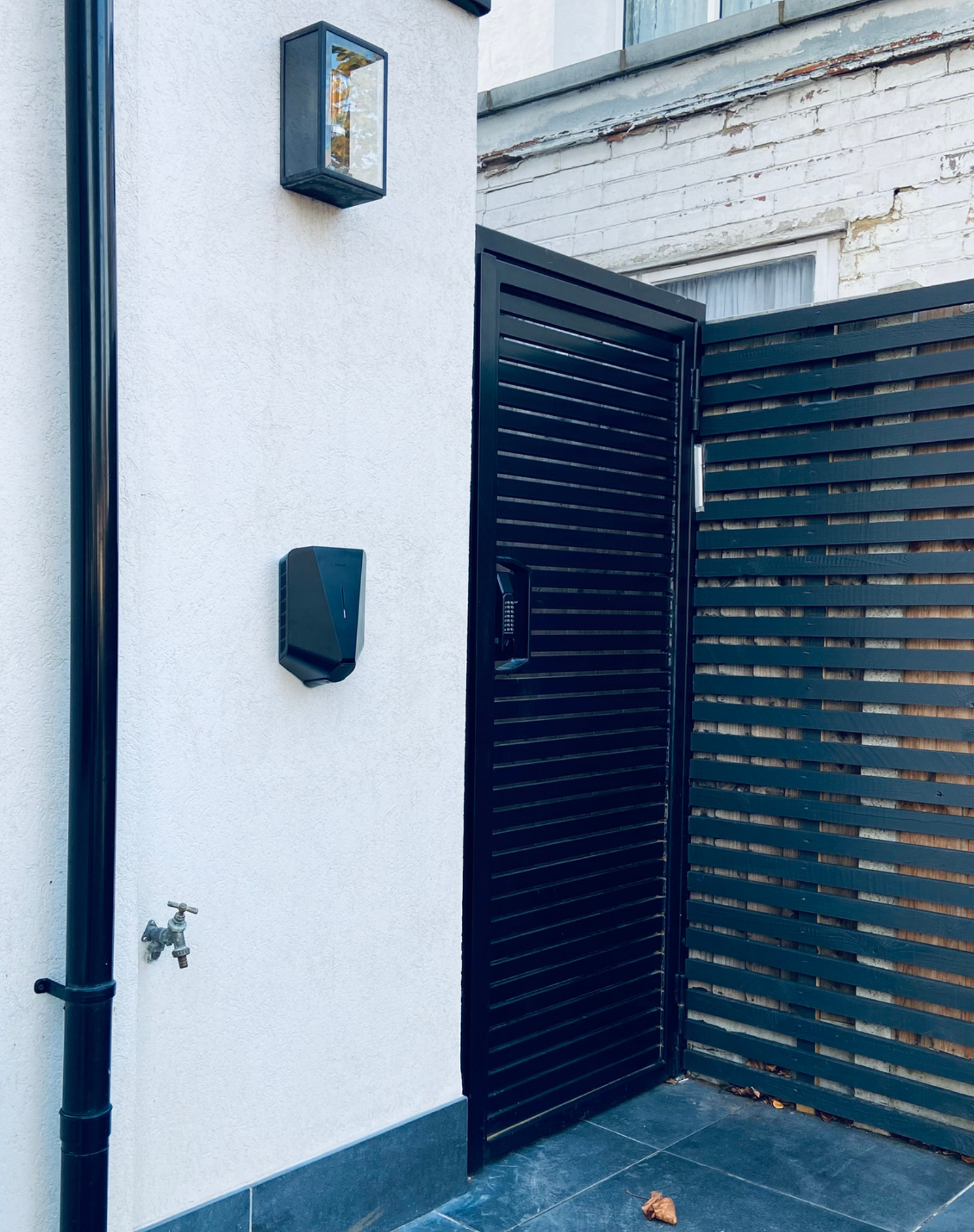
A 7Kw single phase Easee EV charging point is fitting perfectly with the architectural style of this property. The supply cable comes through the wall for a clear result.
